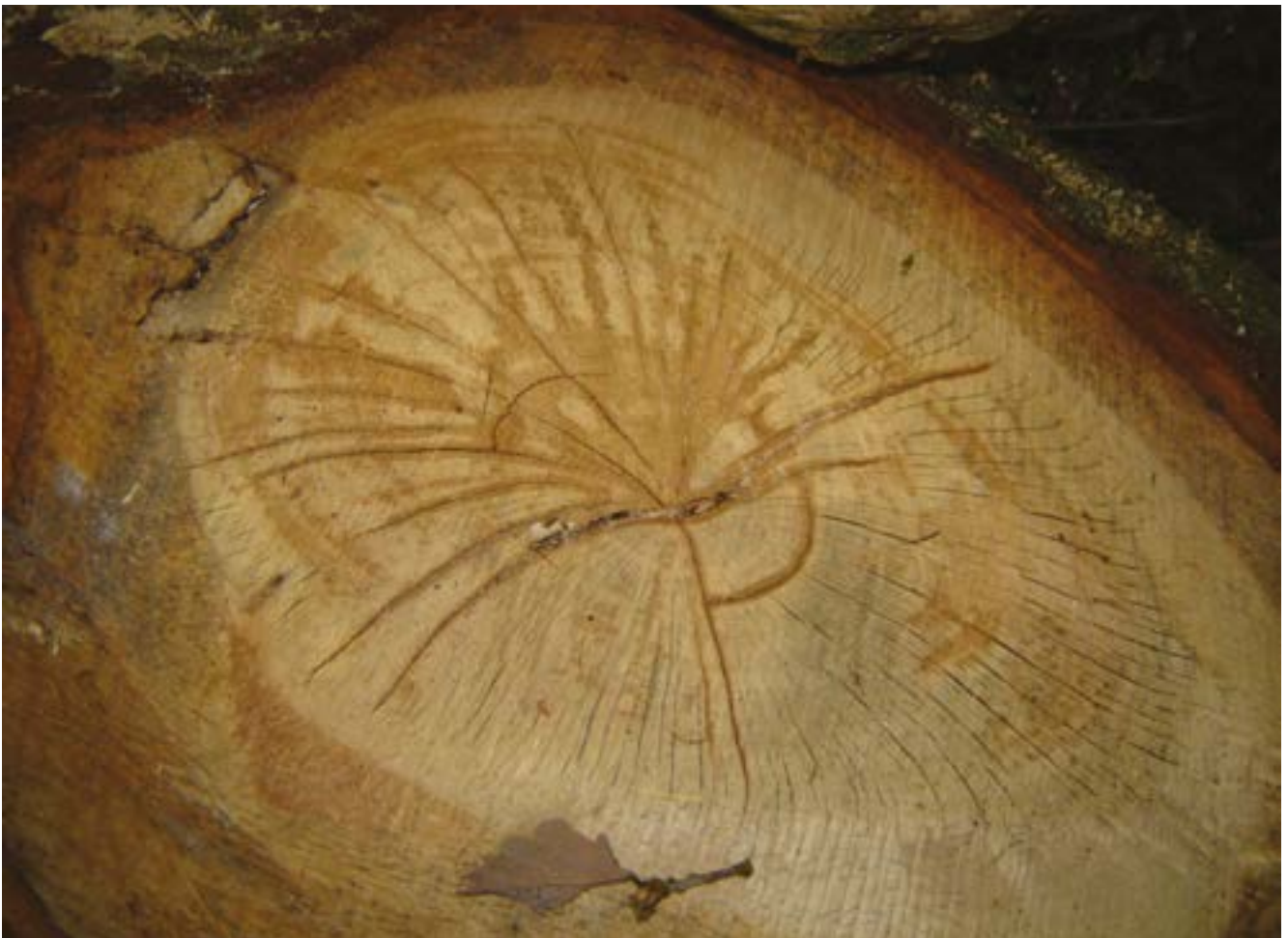
Figure 1 Star and ring shakes present in the same log (the unstained cracks are natural 'checks' caused by the drying-out processes).
